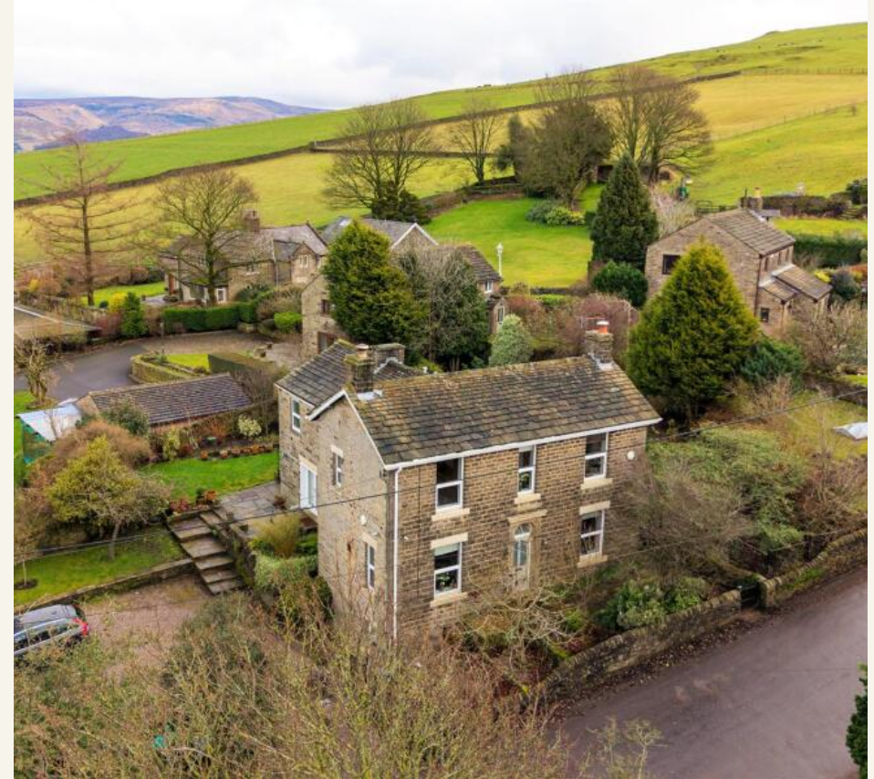
THE FRONTAGE · EASTERLY ELEVATION
